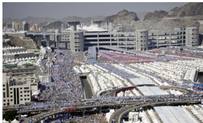
Figure 2: Aljamarat Bridge. Source: Edrees (2016).
